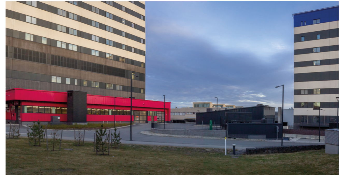
Figure 18. View from Kiviharjunkuja to the southeast.
