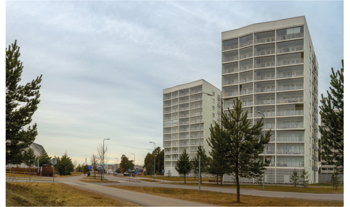
Figure 12. View from Sairaalanrinne to the northwest.
