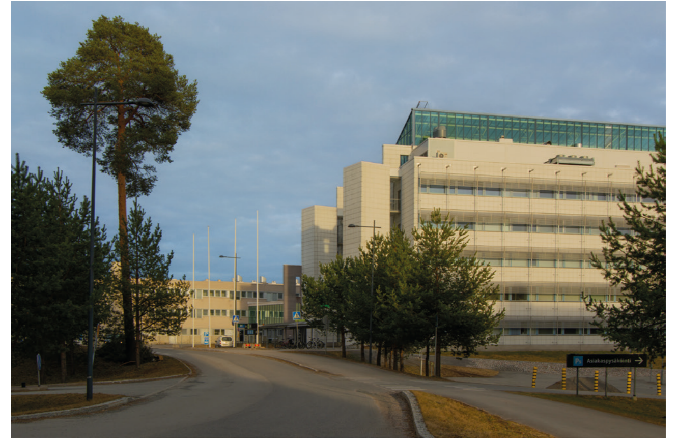
Figure 17. View from Kiviharjuntie to the southeast.
