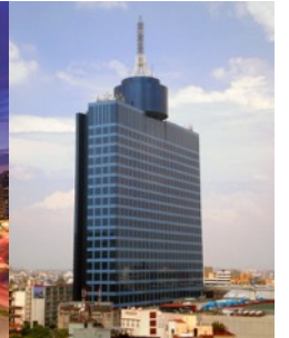
WTC Mexico- torni
