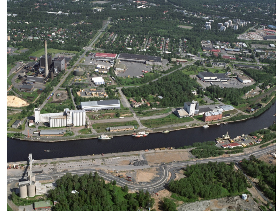
Aerial view A
